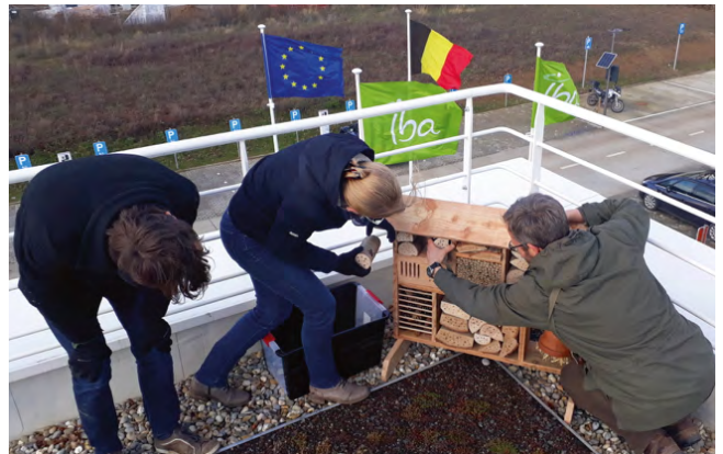
Insect hotel on headquarter’s green roofs
